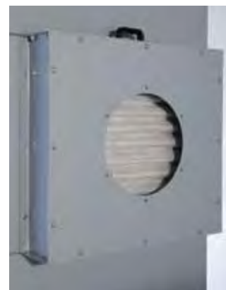
Detail of outside air filter extraction
